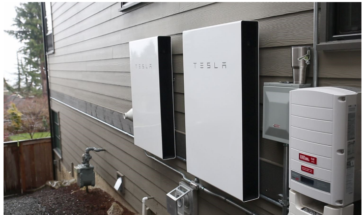
Power wall mounted on the outside of a home.
